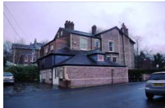
Inappropriate modern annex at no. 78 Ashley Road
