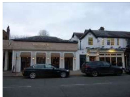
Intrusive stone and timber cladding on an historic building at 169 Ashley Road
