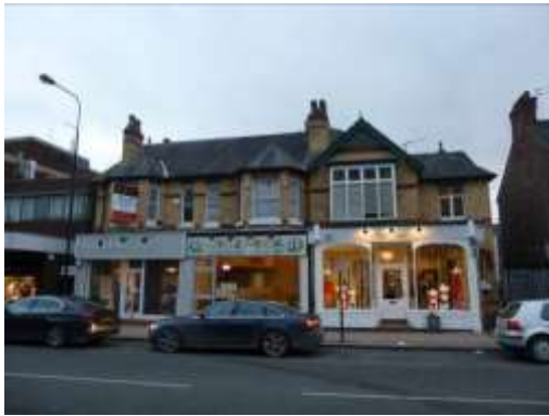
Traditional shop front at 186 Ashley Road (right), next to two inappropriate modern shop fronts (190-188 Ashley Road) with large fascias and aluminium framed glazing
