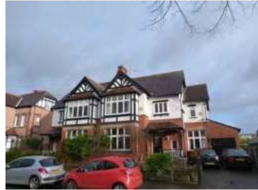
Arts & Crafts dwellings on Heath Road with original boundary walls
