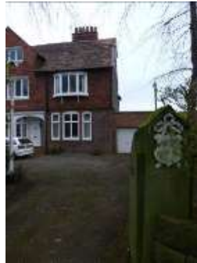
Original stone gate pier at 103 Ashley Road
