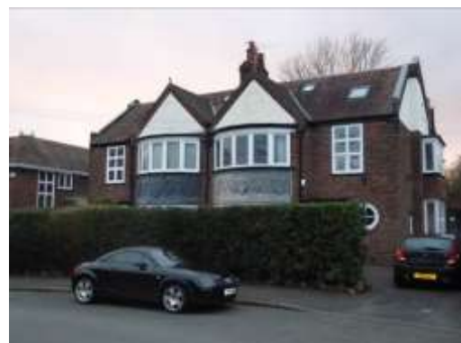
Typical Arts & Crafts materials including textured bricks, decorative plasterwork, clay tiles, casement windows and timberwork
