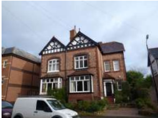
Polychromatic brickwork, rebuilt boundary treatment and a loss of decorative timber detail on the gable end
