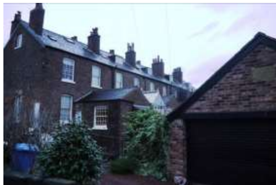
Rear elevations along the residential dwellings of Ashley Road, within Character Zone D
