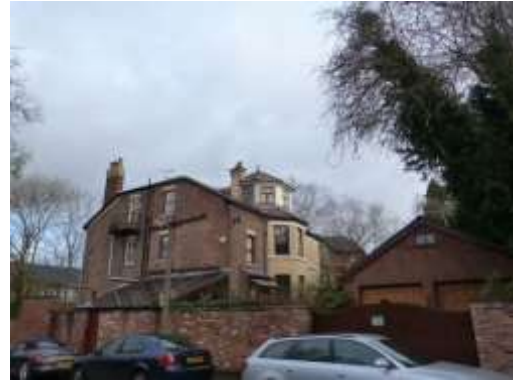
Large property on Heath Road that has potential for enhancement to improve the heritage values/significance
