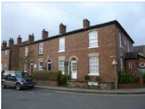
Early 19th century architecture including burnt header bricks, sash windows and simple façades
