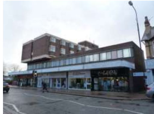
Modern development within the Ashley Road extension (outside the Conservation Area)
