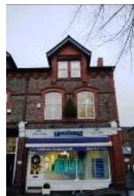
Detail of the late Victorian brickwork including header bond, red brick window surrounds and brick dentilled eaves. The shop front is also original.
