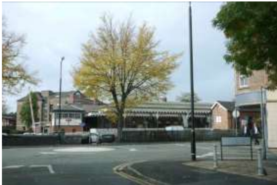
Wide views of Hale Station are a focal point of the Conservation Area
