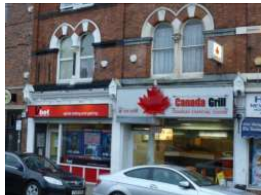
Original shop front capitals, pilasters and façades are dominated by inappropriate back-lit signage in modern materials within Character Zone A
