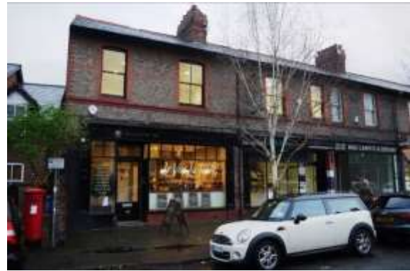
Original shop fronts, designed as part of a short terrace, with pilasters, slender glazing bars and recessed doorways, 4-10 Broomfield Lane
