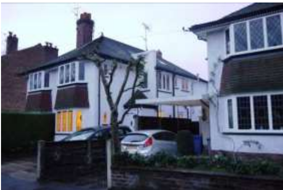
Early 20 th century housing, with original leaded glazing on Spring Road.
