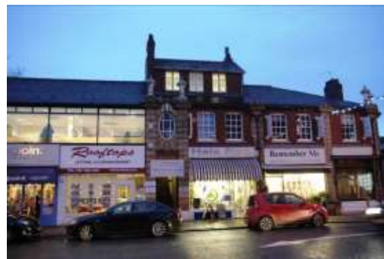
Inappropriate infill development (left) at 161 Ashley Road
