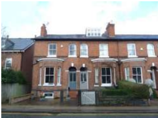
Original low stone wall and planting, with gate pier at number 123 Ashley Road. These have been removed from 125 Ashley Road to create space for parking.
