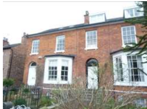
Simple red brick terraces, bay windows and 6 over 6 sash windows in
