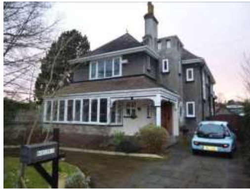
Note the original leaded windows on the ground floor and the original external pebbledash
